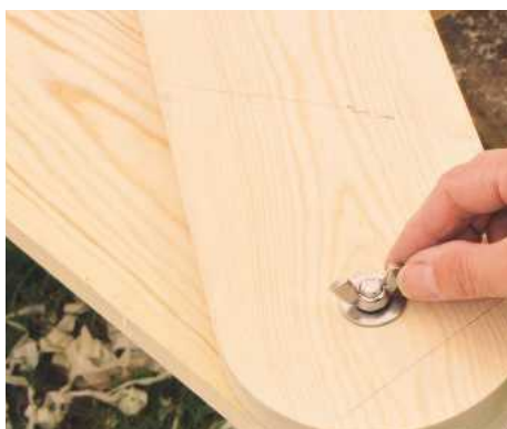
14 Check that front and rear uprights line up and coach bolts fit snugly, then secure with washers and wing nuts
