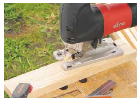
3 Cut a bevel on end pieces with a jigsaw or bandsaw, taking care to keep on the waste side of the pencil line
