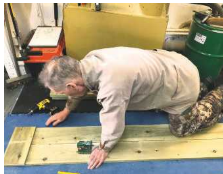
Constructing one of the filming area panels
