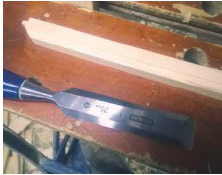
44 Using chisels (or a router), cut a rebate on each piece that the compartment can slide into
