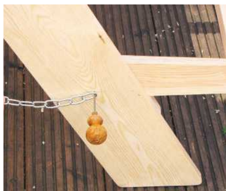
25 To prevent uprights opening out too far, fix galvanised chain both sides, experimenting with its position
