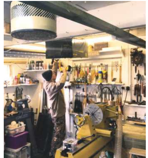
Fixing some of the materials in place
