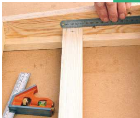
19 Each shelf tray has five slats; the centre one is nailed, with others left loose for plant pot drainage
