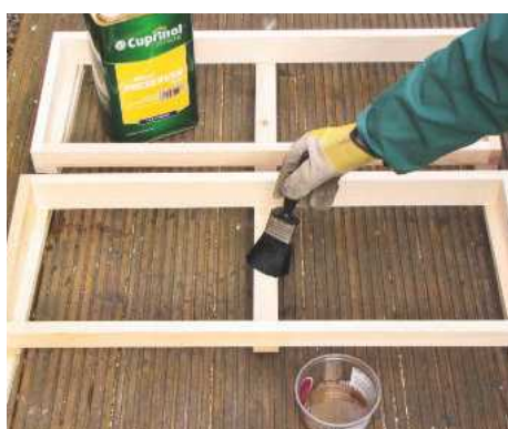
28 Treating all timber with suitable clear preservative, such as Cuprinol, will extend the planter's life
