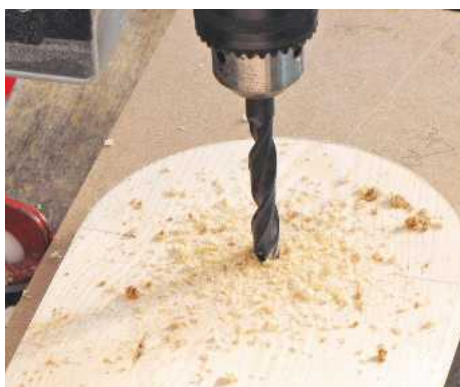
13 Carefully drill a 10mm-diameter hole to suit a coach bolt; repeat process on both rear uprights
